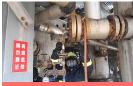
Repair team stops leakage and repairs damaged equipment
